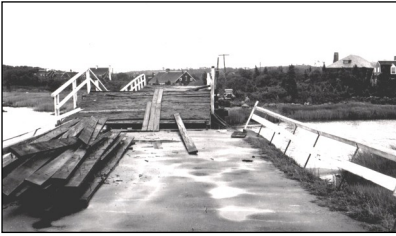
Bridge on Chapoquoit Road, 1938.
